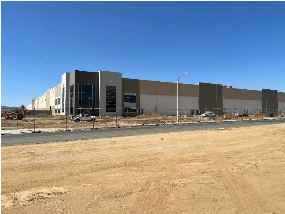
Photo 8 – View showing industrial building under construction to the south.
