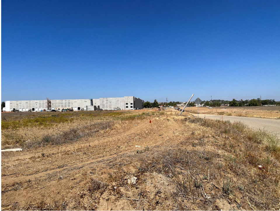
Photo 1 – View from northeastern corner of Property towards the west.
