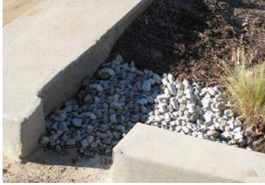
Figure 2: Curb Cut located in a Bioretention Facility
