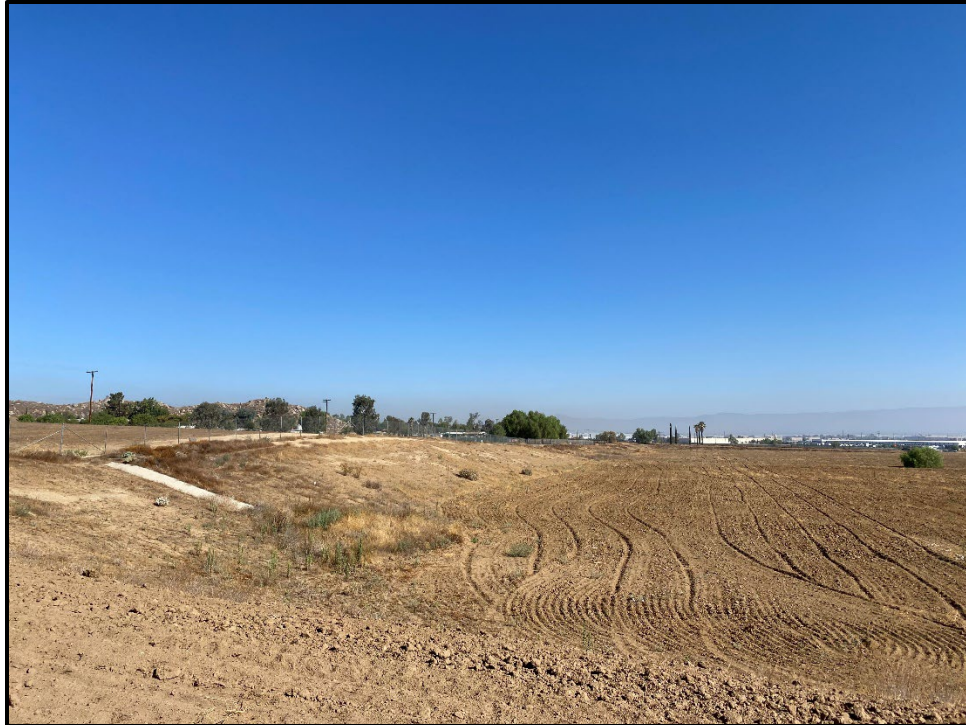
Plate 4.2–1: Overview of the project, facing north.
