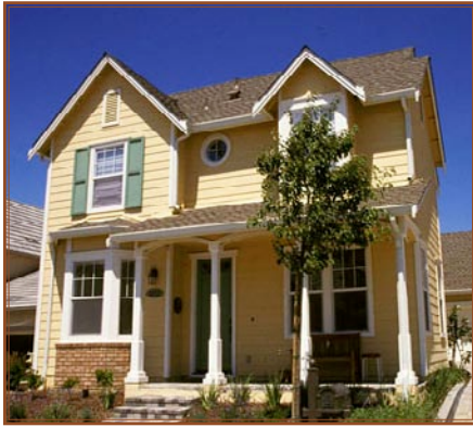
Porch, Posts, Materials and Roof Form
