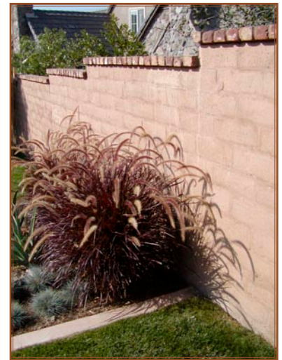
Community Perimeter Wall
