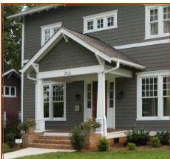
Gable Porch with Columns as Main Elevation Feature; Simple Brackets
