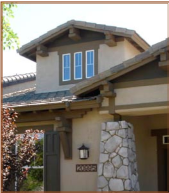
Exposed Rafter Tails and Materials
