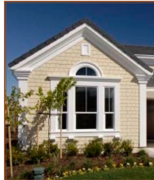
Boxed Eaves and Pedimented Window
