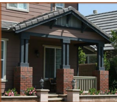
Double Posts on Piers
