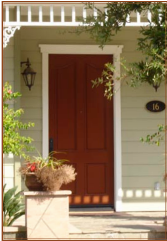
Contrasting Wood Trim Around Doors
