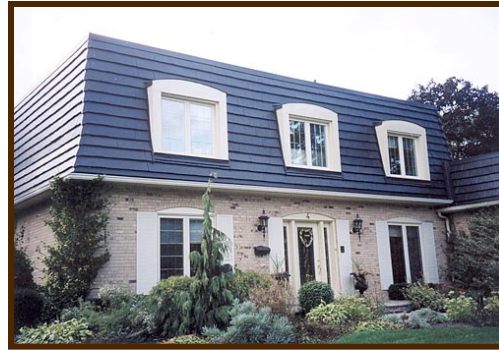
Inappropriate Design: Example Mansard Roof
