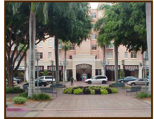
Example of Pedestrian Walkway
