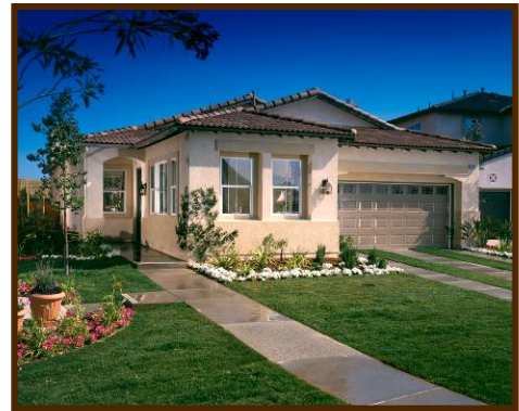
Example of Mid-Recessed Garage.
