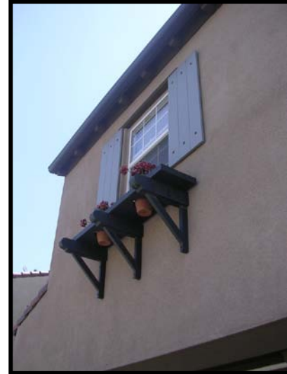
Figure 5-7 Example of pot shelf under window
