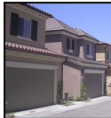
Figure 5-12 Landscaping planters next to garages
