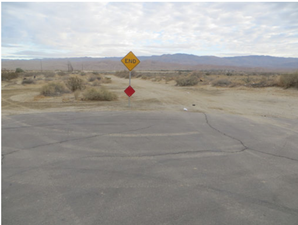
Photograph 4: From the northern terminus of Cook Street looking north along the alignment and existing dirt road.
