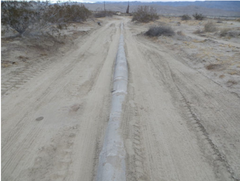
Photograph 3: Existing pipeline within the existing road right of way in the undeveloped northern portion of the distribution alignment.
