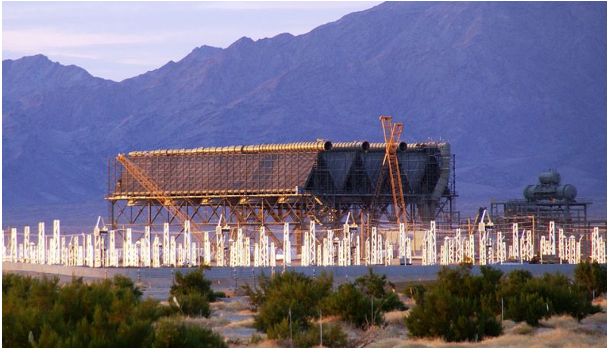
Air-cooled condenser under construction at the Genesis solar project in Riverside County, outside Blythe, California.
