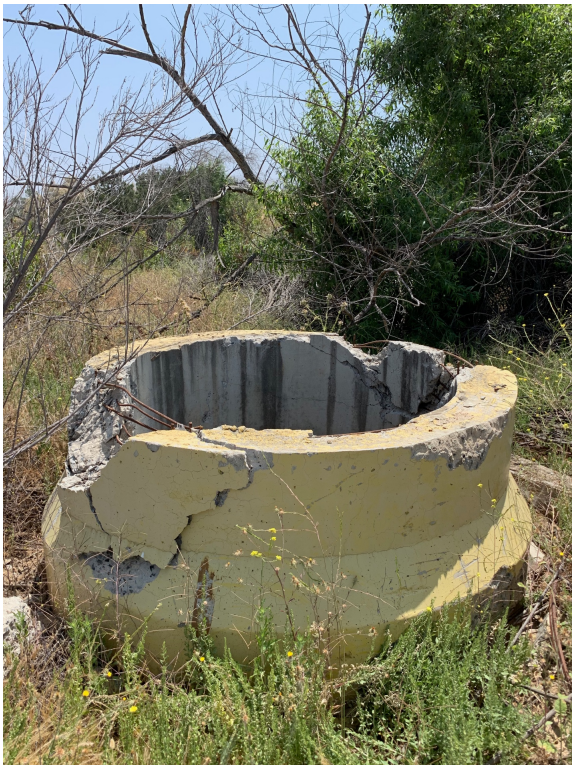
Figure 19 Top of manhole
