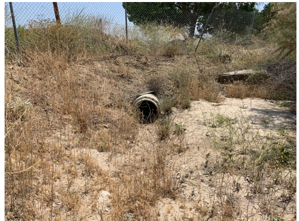
Figure 20 Concrete pipe at the NE corner of the Site
