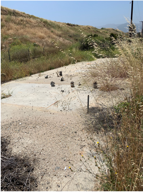
Figure 21 Former electrical equipment pad along the southern border
