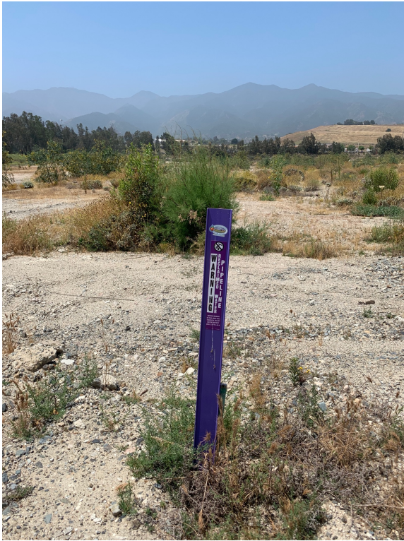
Figure 17 Reclaimed water marker at the Site
