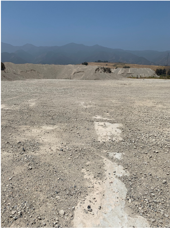
Figure 13 Concrete from former plant foundations
