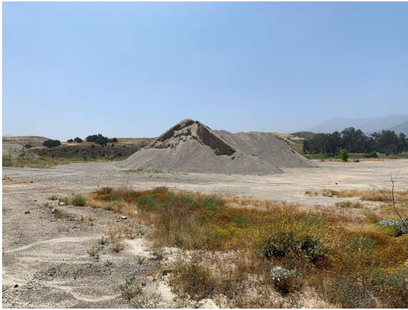
Figure 9 Crushed concrete pile in former plant area
