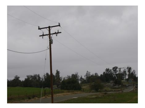
**Photograph 8:** Southwestern view from APN 314-020-017 of one pole-mounted electrical transformer located along the southern perimeter of the Subject Property.
