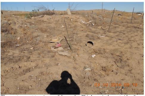
The westernmost terminous of the swale. This berm is the east side of Decker Road. This structure has completely isolated the swale from receiving upstream hydrology.
