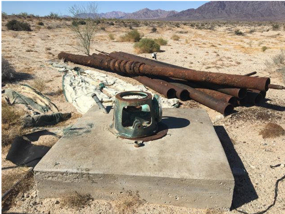
AREA A: View of irrigation well and removed casing in the northwest portion of Area A.
