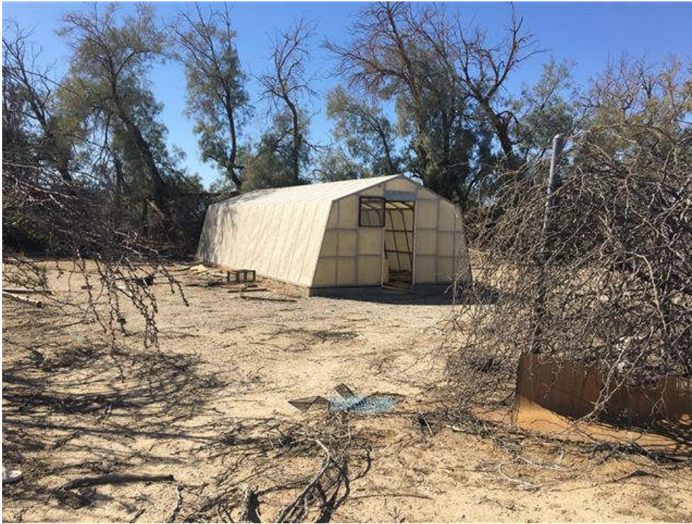
AREA A: View of greenhouse in the west-central portion of Area A.
