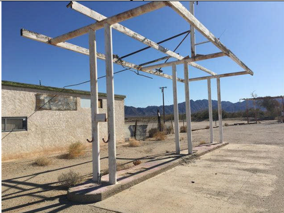
Adjacent Land: Former gasoline station along Rice Rd (SR-177) that is adjacent to the west of Area B.
