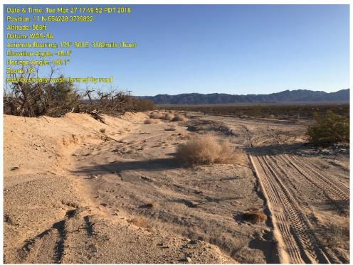
**Photo 4** – Parcel Group A. Eastern boundary facing south. Earthen berm on east boundary directing flow down perimeter road. Flow emanates from fallow agriculture field with windrows upslope.
