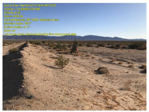
Photo 1 – Parcel Group A. Northwest corner facing south. Earthen berm intact. Distal extent of Pinto Wash diverted along the western boundary.
