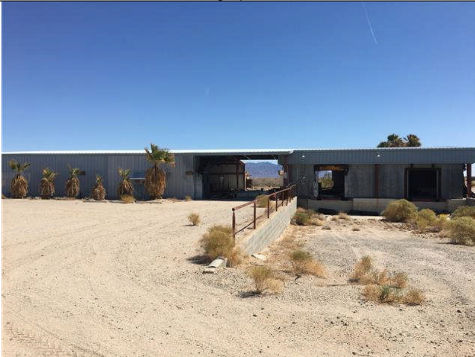
AREA B: View of former packing house in the southwest portion of Area B.
