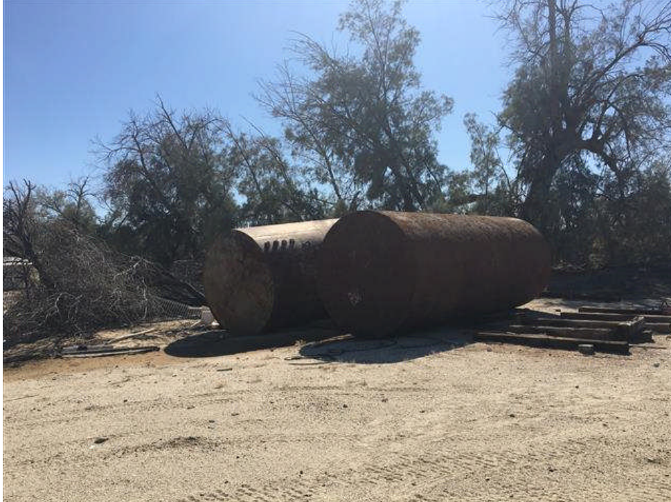
AREA A: View of fuel ASTs in the west-central portion of Area A. They appeared to currently be unused.
