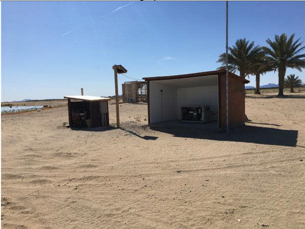
AREA F: View of generator shed north of the residence in the central portion of Area F. No staining or evidence of a release was observed.
