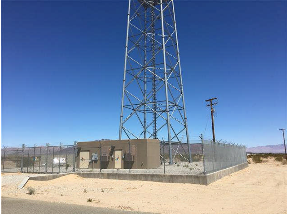
AREA B: Facing north toward the gen-tie line segment that connects to Area A (as shown in Photograph 8)
