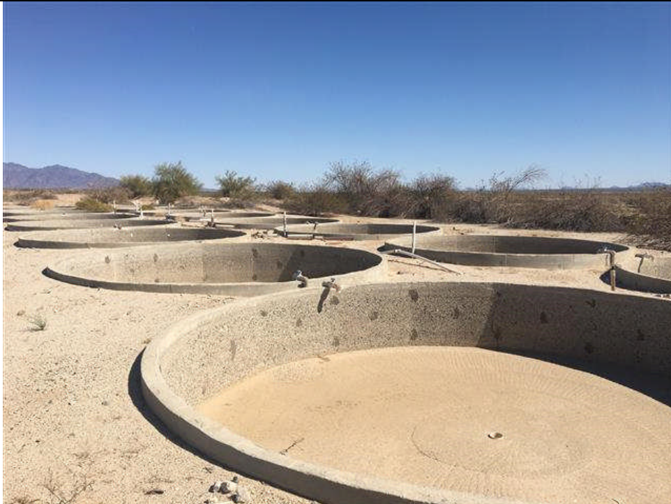
AREA A: Concrete fish tanks in west-central portion of Area A.
