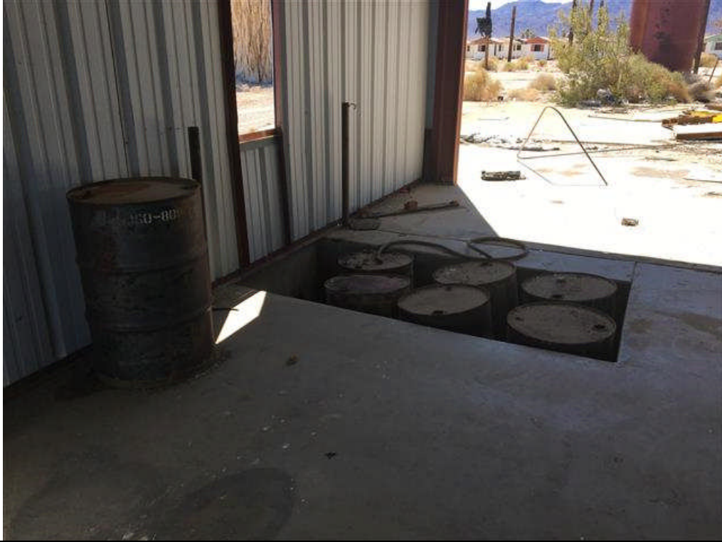
AREA B: View of sump with 55-gallon drum storage.
