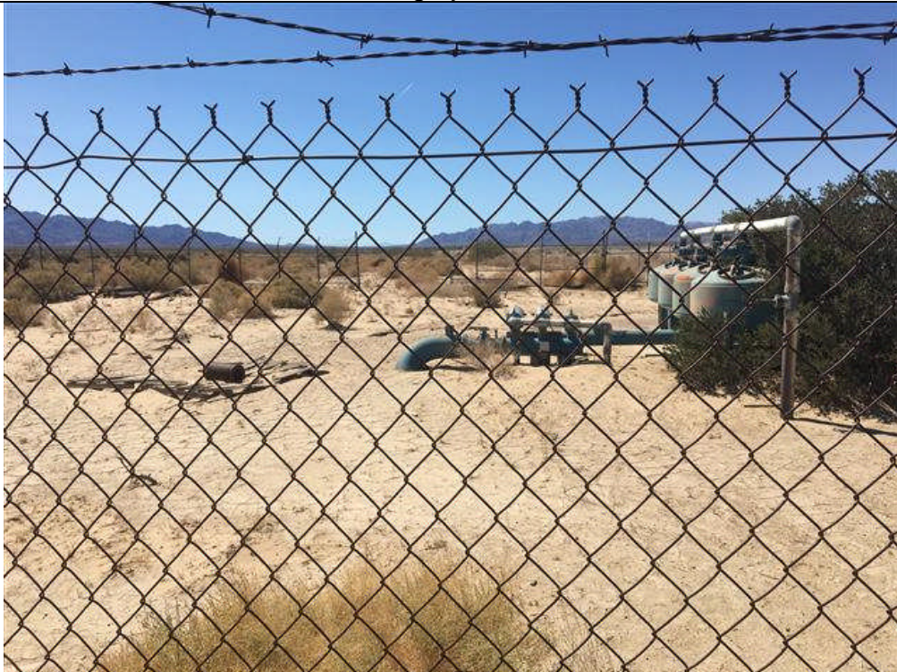
AREA D: Irrigation well near the northern boundary of Area D.
