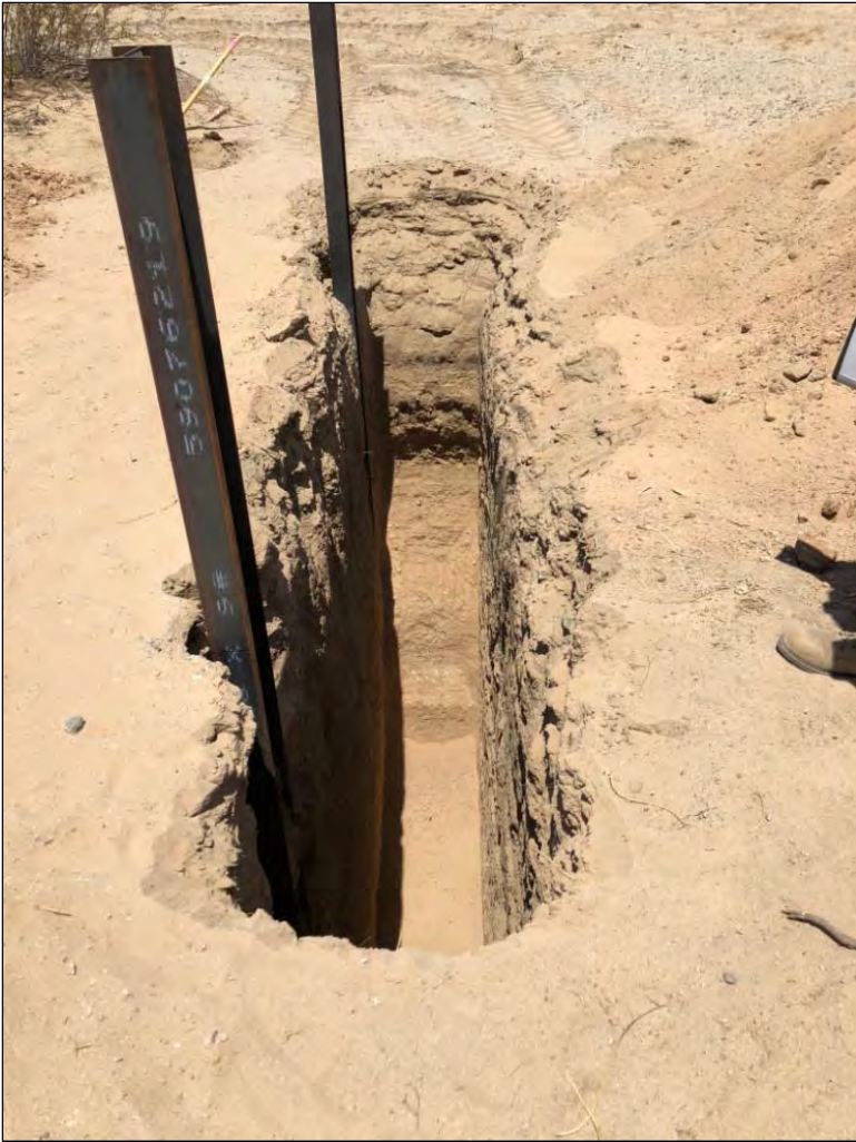
Figure 6-8 Example of excavated geotechnical trench (TP 17, facing west).
