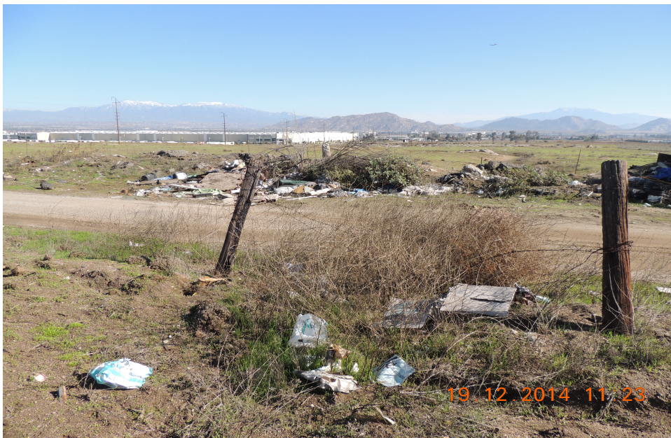
Intersection of Decker Road and remnants of the swale.
