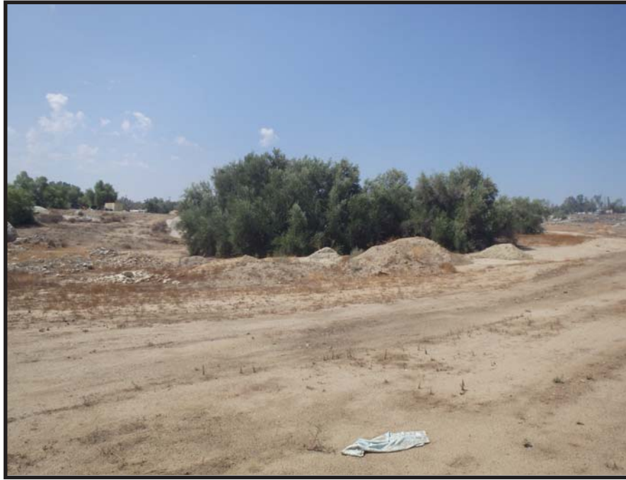
PHOTOGRAPH 5 - Southwestern view from southwestern region of APN 314-040-001; olive trees are found onsite in two locations.
