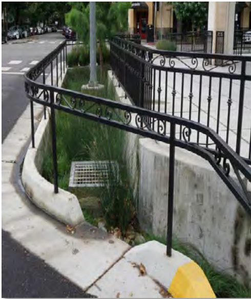
Figure A: Urban Infiltration Trench BMP
