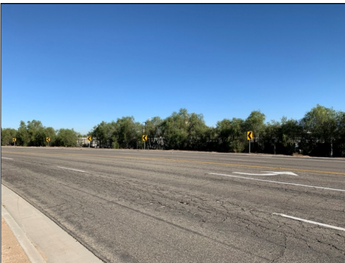
41. Harvill Avenue and the adjacent properties to the east, view facing northeast.
