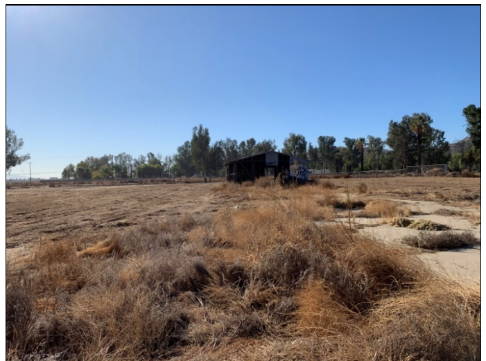
36. Foundations north of the former building on the northwest portion of Parcel A, view facing southwest.
