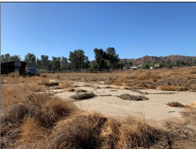
35. Foundations north of the former building on the northwest portion of Parcel A, view facing southwest.
