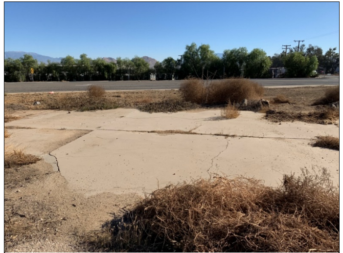
4. Foundations on the southeast portion of Parcel B, view facing east.
