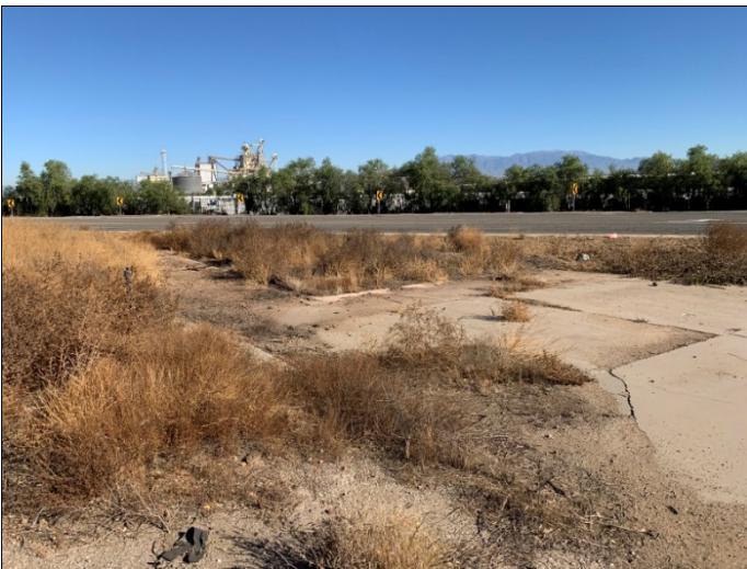
5. Foundations on the southeast portion of Parcel B, view facing northeast.
