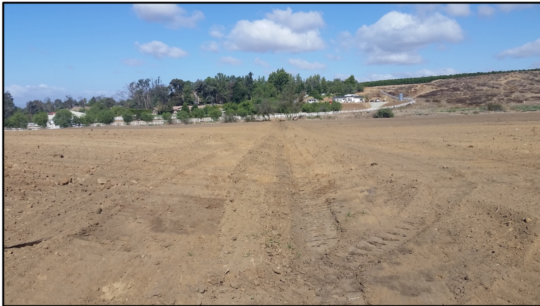
Plate 4.2-2: Overview of the northern half of the project, facing west.
