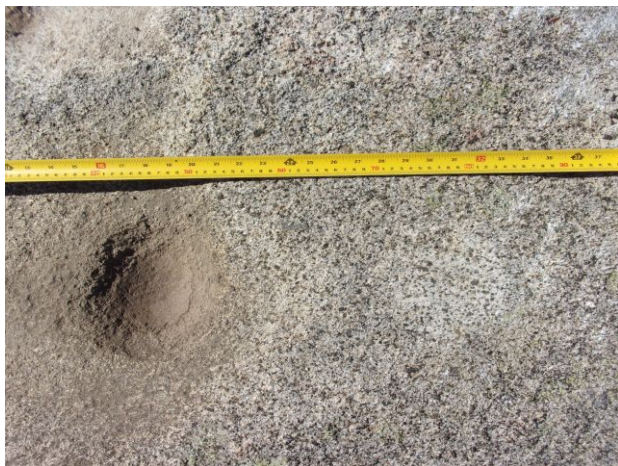
Photograph 21. MMJC-1 mortar and slick basin detail (Oblique)
