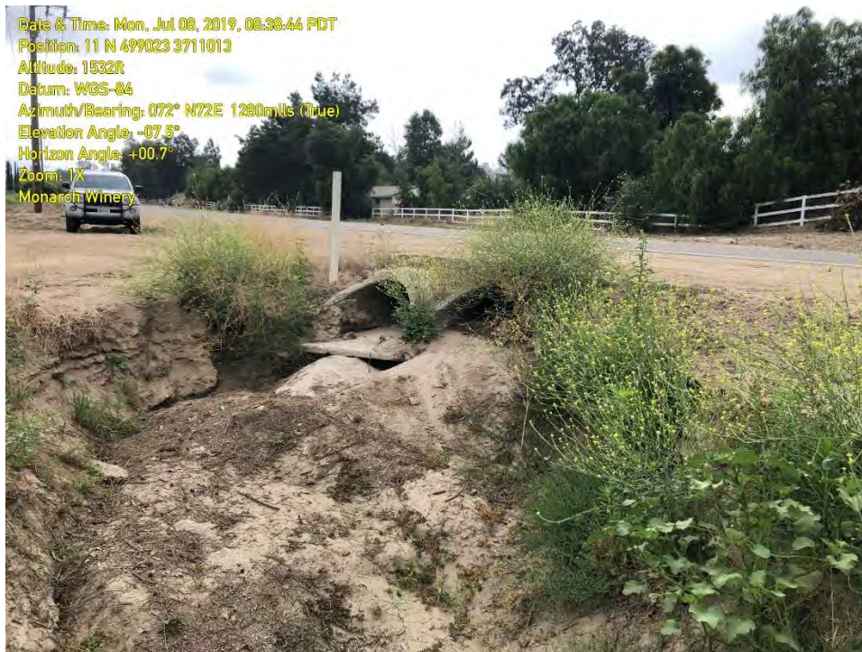
PHOTOGRAPH 4: The two 24-inch culverts convey flows into a small collection area near the Site's entrance.
