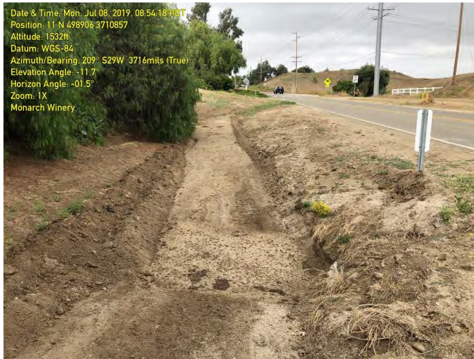
PHOTOGRAPH 9: Human-created channel leading into the single 24-inch culvert on the eastside of De Portola Road.
