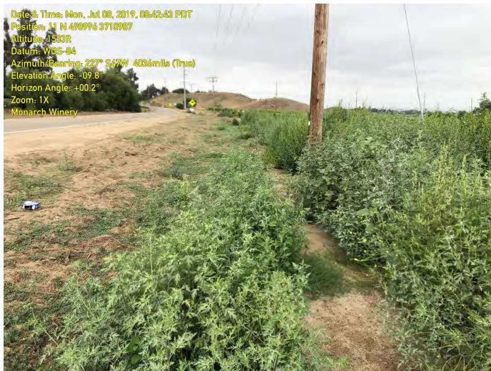
PHOTOGRAPH 5: No clear roadside drainage or Riverine feature was present downstream of the culvert conveyance area indicating flows dissipate to sheetflow.
