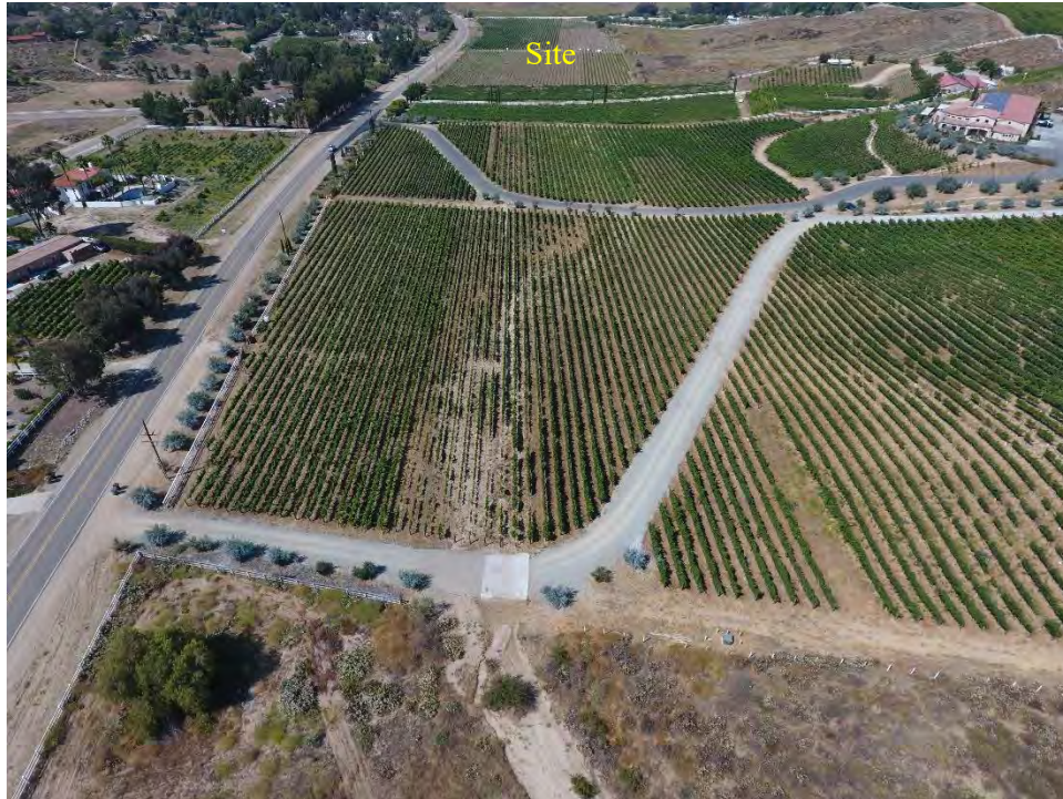
PHOTOGRAPH 1: A view of Long Valley Wash upstream of the Site. The “natural” wash enters a vineyard where flows still appear evident.
