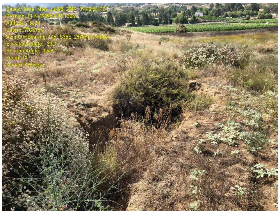
PHOTOGRAPH 20: A view of the erosional gully farther downstream.
