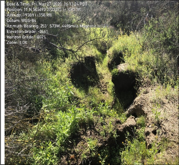
PP 7 looking west (D 1a)
