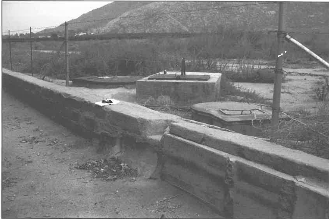
Image053.jpg: View of access port near SMO-4 site. Manhole for the conduit is located in the square vault. From this point the conduit runs beneath the orchard (off to the left). The orchard in Image014 is located in the far background. In the foreground, mounded earth can be seen beneath high brush. This represents the earth cover for the conduit. Port noted as #2 in archival photo below.
