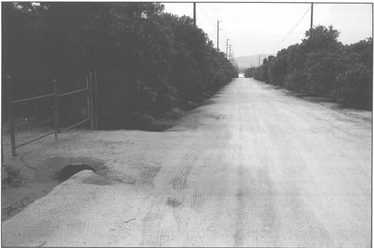
Image057.jpg: View southwest of the site near eastern end.
