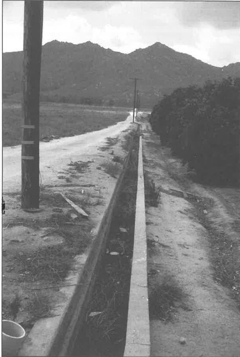
Image016.jpg: View of northern end of site to the south showing Feature 3, a retaining wall and concrete runoff-only flume located in the southern half of the site.
